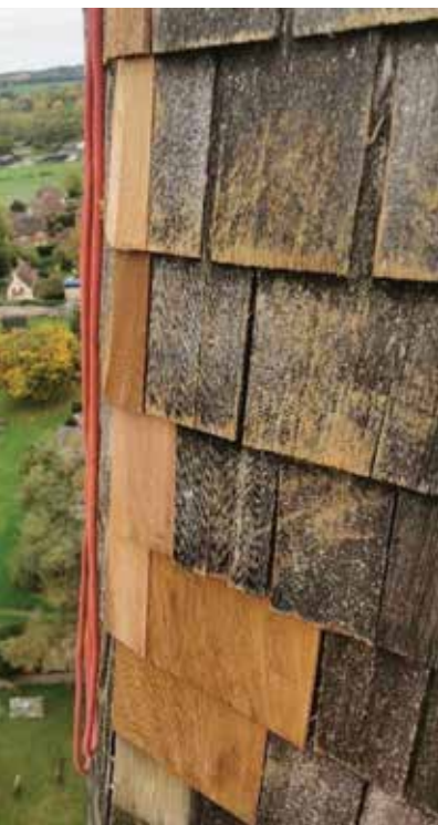
Patching decayed shingles on the spire at Brimpton
