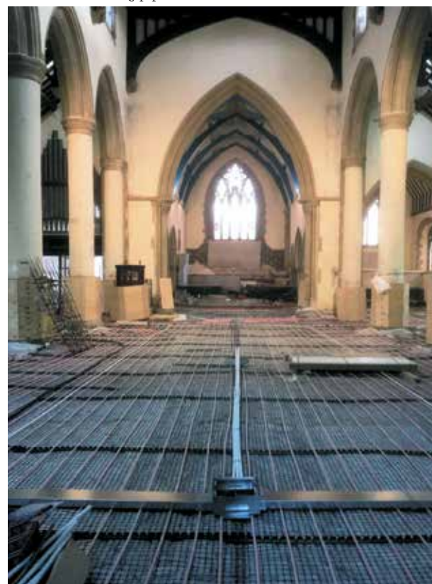
Underfloor heating pipes and electrical service ducts
