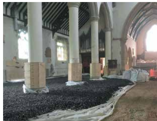
The black material is an insulation layer of recycled glass
