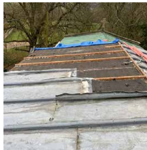
Combe - the roof after previous theft of lead
