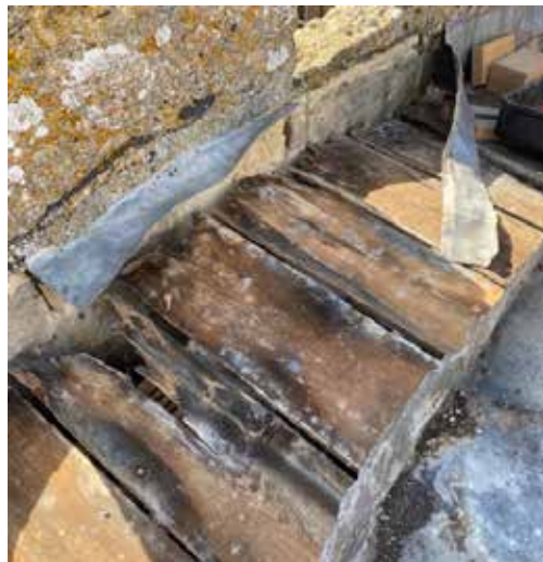
Decayed roof timbers on the tower at Farnborough
