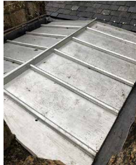
East Garston - the porch roof, with new oak rafters covered with terne-coated steel to replace the stolen lead
